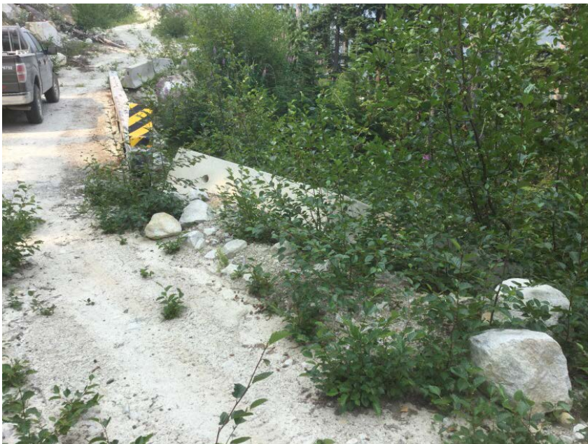
Downstream right approach barriers
