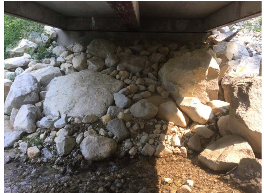
Right Bank Abutment when facing downstream
