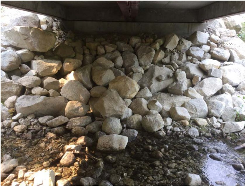
Left Bank Abutment when facing downstream
