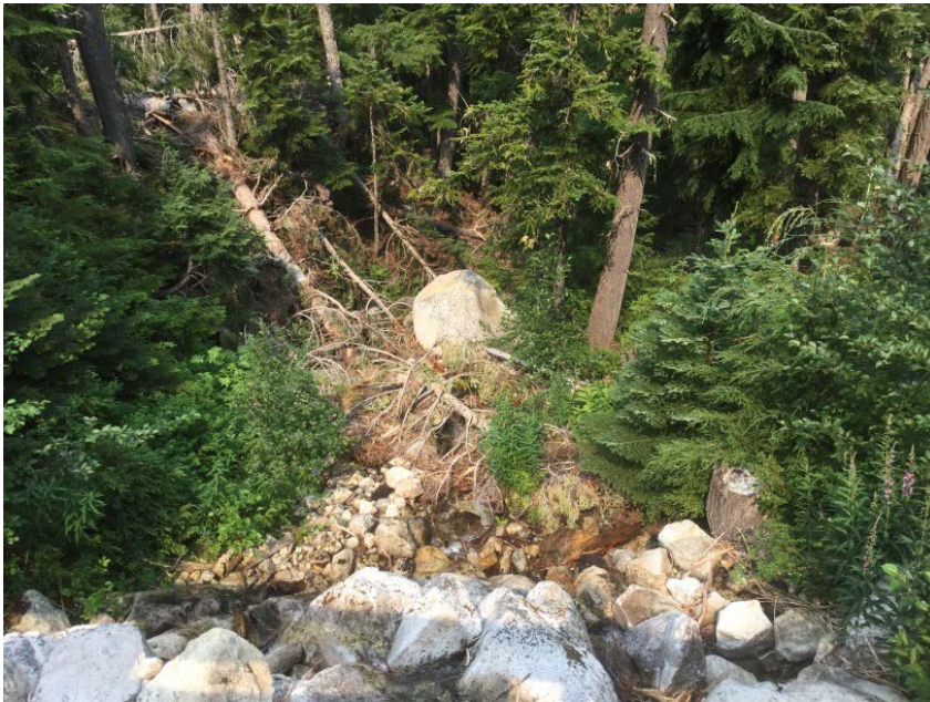
Looking downstream from deck
