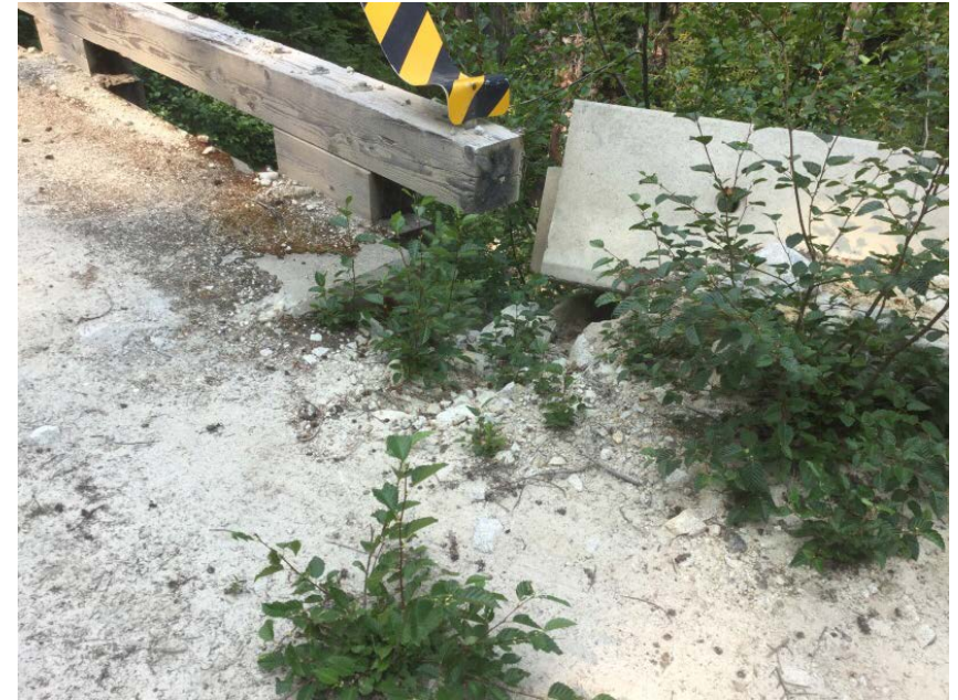
Downstream right approach fill
